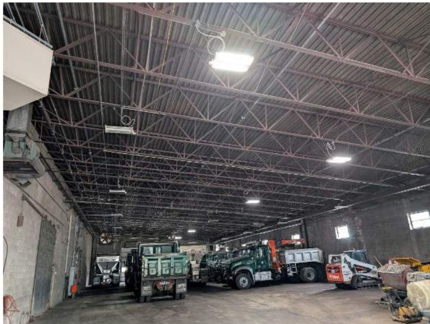
Photo: Steel joists and roof deck framing into load-bearing CMU walls
