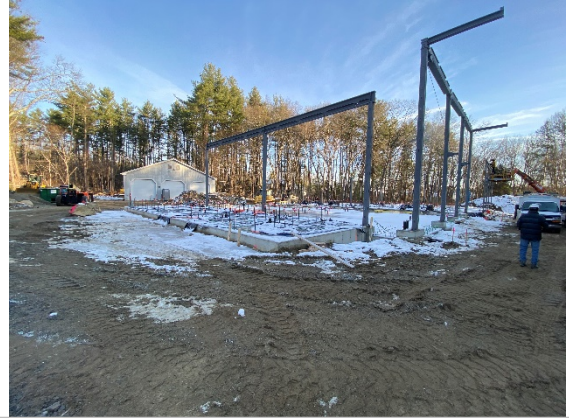
Erection of steel framing (12/11/2020)
