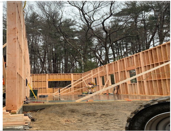
Interior and exterior wood framing installation (12/31/2020)
