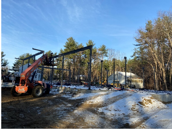
Erection of steel framing (12/11/2020)
