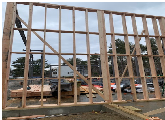
Interior and exterior wood framing installation (12/31/2020)
