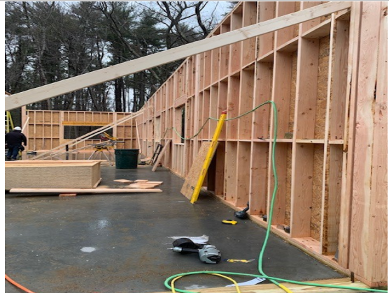
Interior and exterior wood framing installation (12/31/2020)
