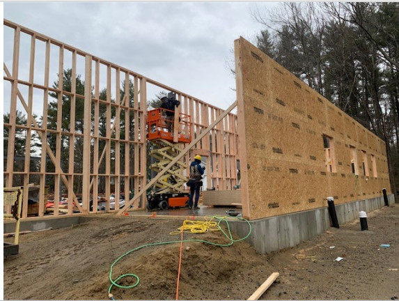
Interior and exterior wood framing installation (12/31/2020)
