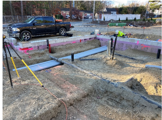
Installation of underground electrical conduits (11/18/2020)
