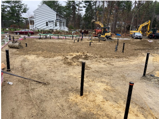
Underground plumbing installed (11/13/2020)
