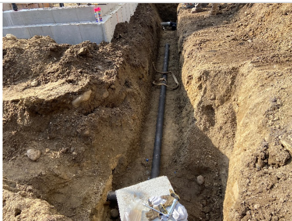
Installation of water main on north side of building (11/20/2020)
