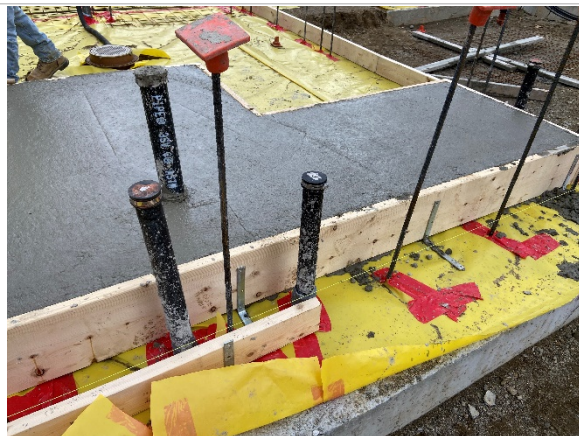
Installation of the 14-inch slab in decon/laundry room (12/02/2020)
