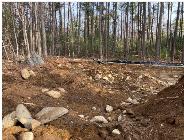
Excavation for detention basin on north side of site (12/04/2020)
