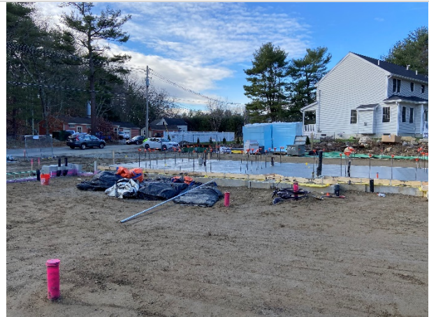
Slab on grade installed on west side of site (12/04/2020)
