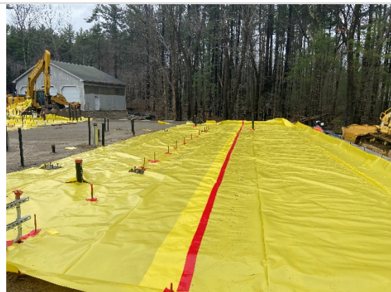
Installation of vapor barrier (12/01/2020)
