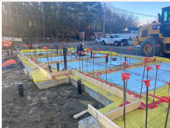
Installation of floor drains (12/02/2020)
