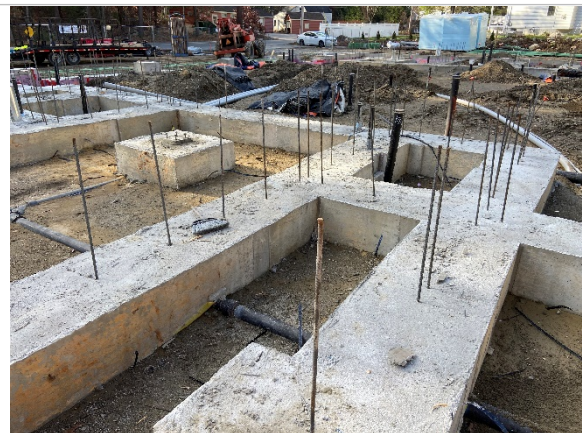
Installed interior foundations (11/24/2020)
