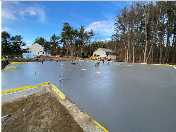
Slab on grade installed on east side of site (12/04/2020)
