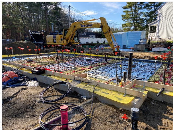
Installation of radiant heating in slab west of apparatus bay (12/03/2020)
