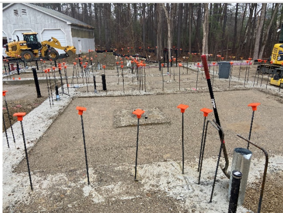
Backfilling of interior to slab subgrade (11/30/2020)
