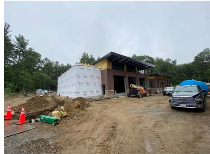
Overview of building from southwest
