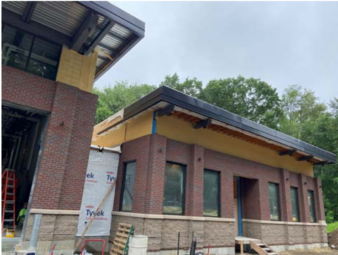
Overview of main entrance
