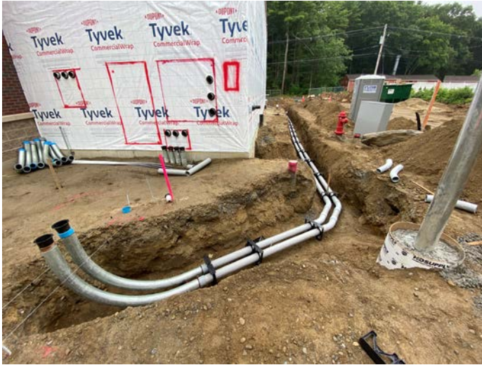
Installation of underground conduit for transformer
