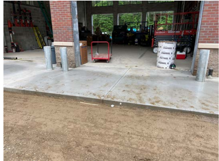
Overview of north side apparatus bay apron
