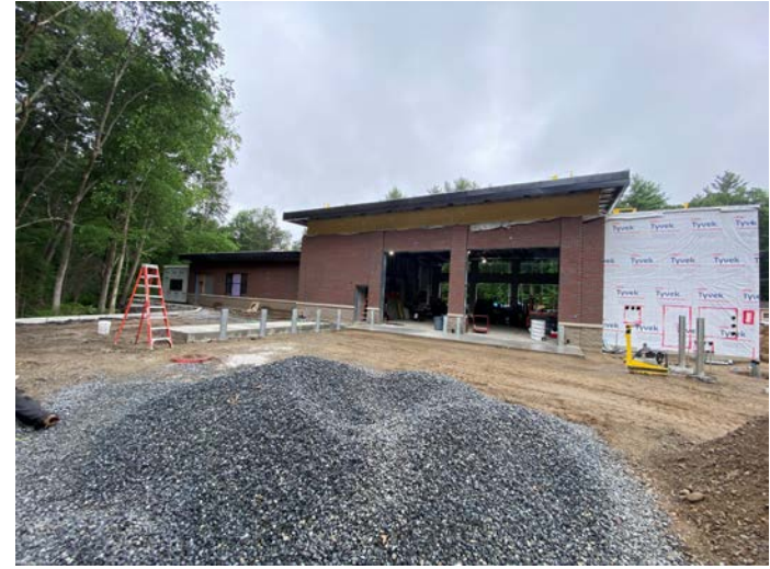
Overview of building from north
