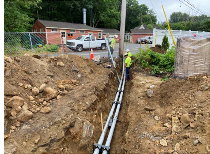
Installation of underground conduit for transformer
