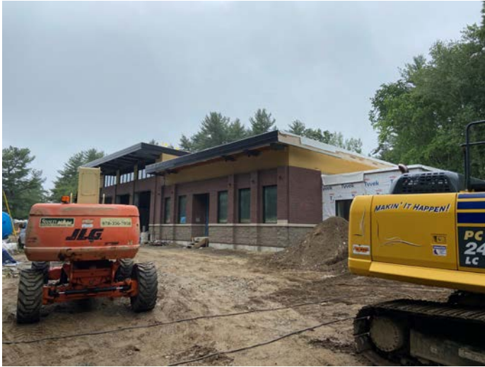
Overview of building from southeast
