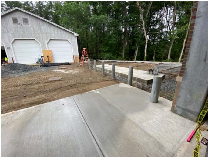
Overview of generator pad and north side apparatus bay apron
