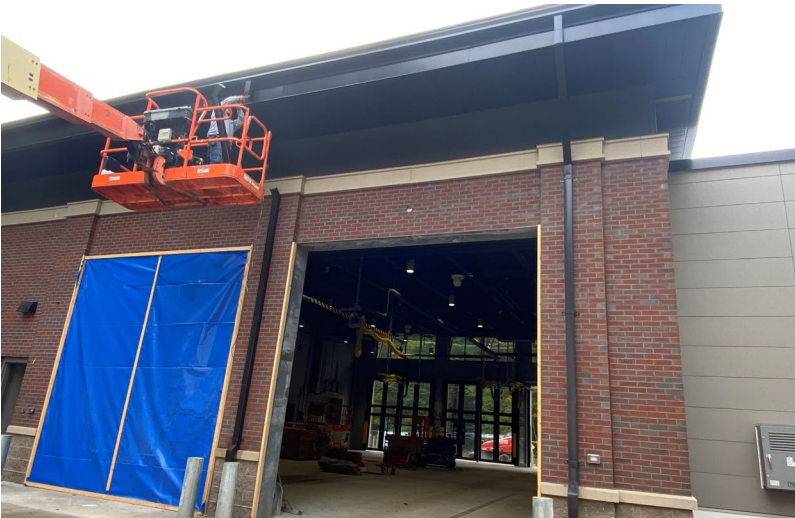
Roof flashing installation
