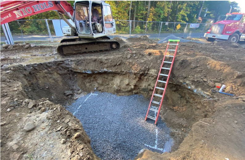
Septic tank excavation
