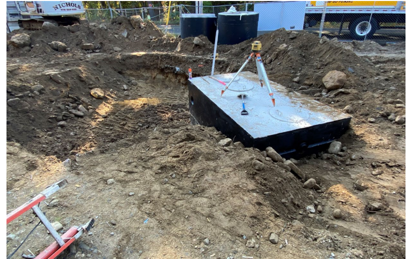
Septic tank installation
