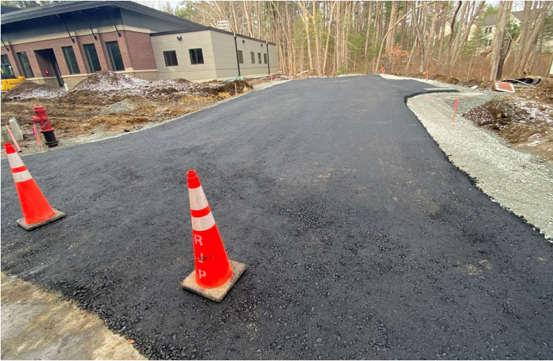
Base paving east side of building
