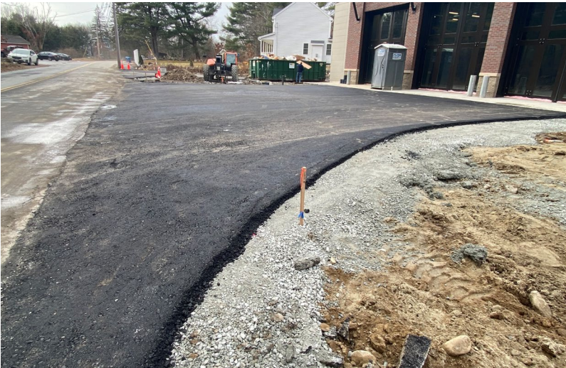
Base paving front of building
