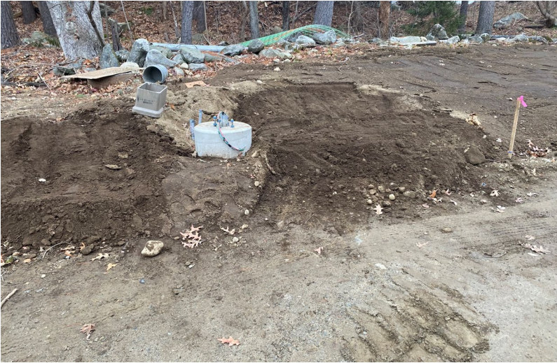
Light pole bases installation
