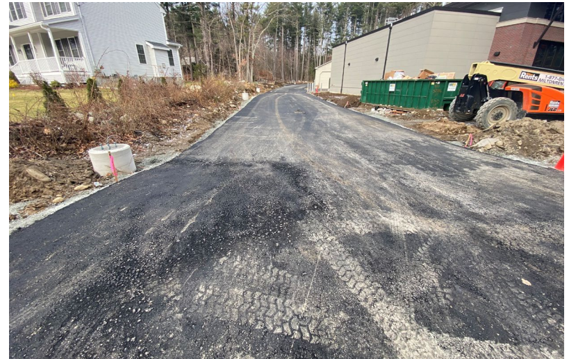
Base paving west side of building
