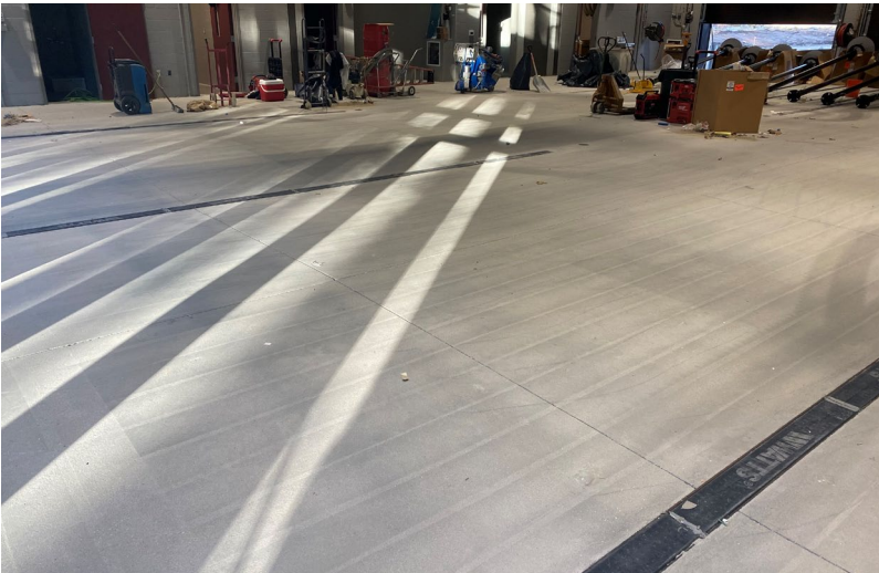
Preparation for epoxy flooring
