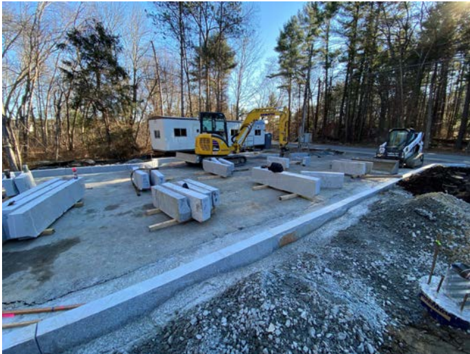
Installation of granite curbs
