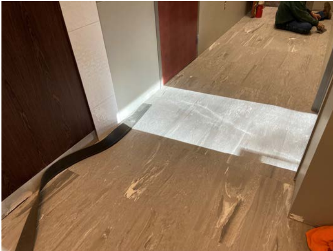
Flooring installation in Corridor 102
