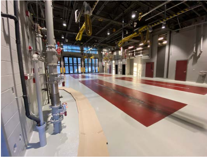
Epoxy floor installation in apparatus bay
