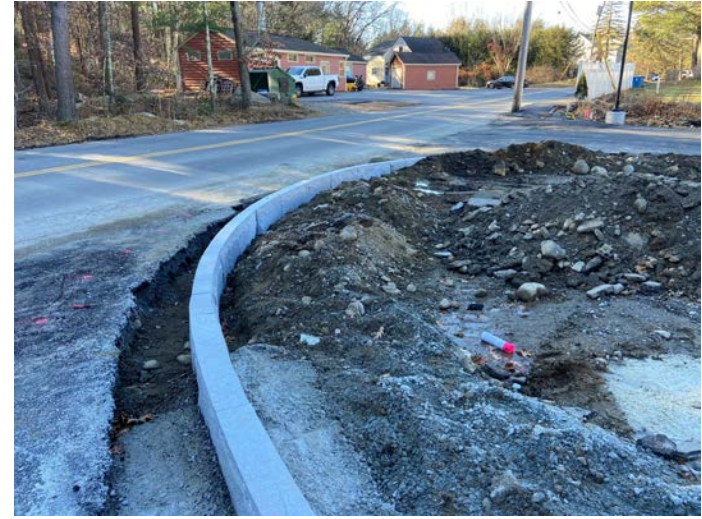
Granite curb installation at southwest side of site
