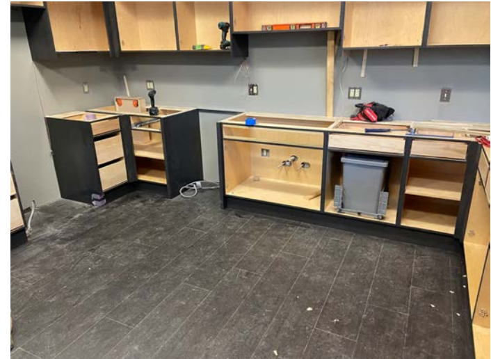
Kitchen cabinet installation
