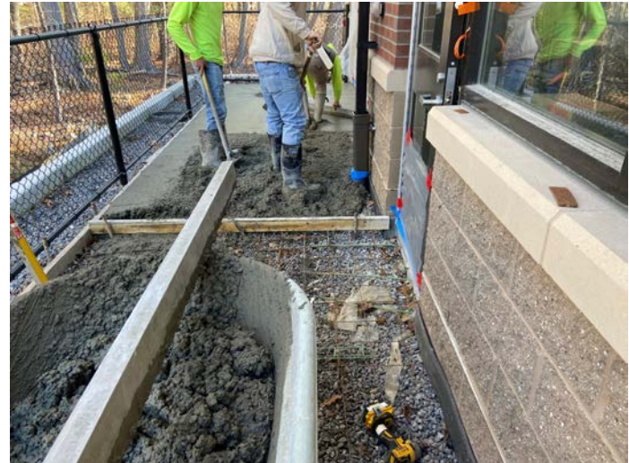
Partial installation of sidewalk on north side of building
