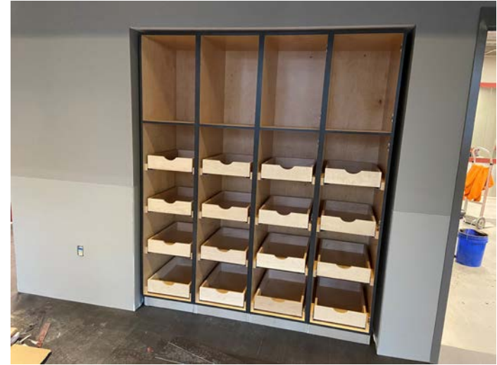
Installation of cabinets in dayroom
