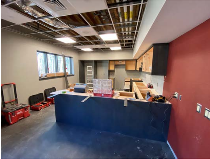
Installation of kitchen cabinets
