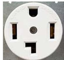
Typically, the 230V outlet where you park at home will be a NEMA 14-50 (same as an electric range) or a NEMA 14-30 (same as an electric dryer). (There are other styles of plugs, but they are less common.) Level 2 chargers come in models from 20 to 50 amps. Some chargers even have adjustable current draw.
