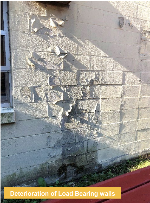
Buckling of Exterior Load Bearing Walls
